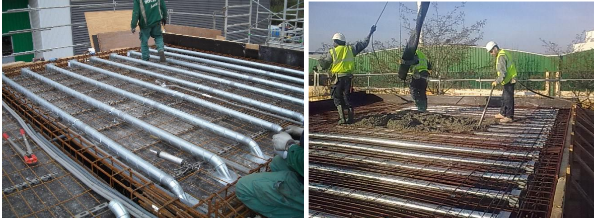
Figure 1: Photographs of the ventilation ducts before and during concrete pouring.
