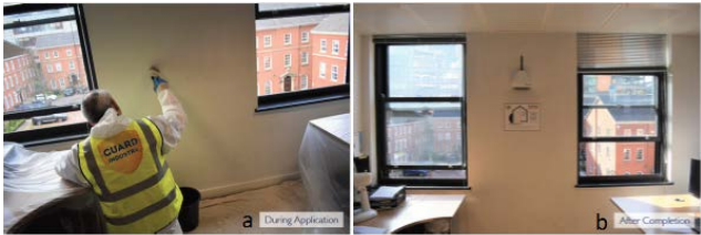
Figure 3. (a) Application of DToxGuard ® Int by brush and windows opened; (b) After completion: the AQMesh ® air quality monitor was setup on the treated wall
