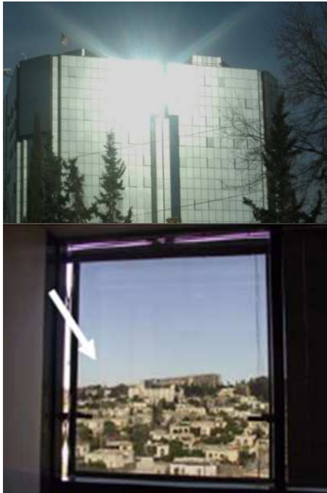
Figure 4. The case study building from the outside (above) and the inside (below)
