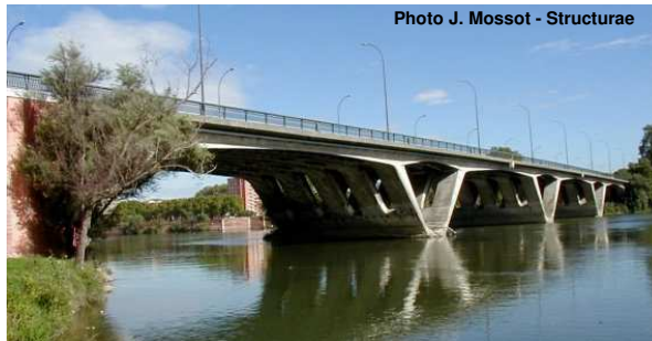
Photo J. Mossot - Structurae
