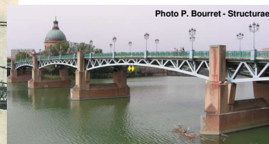
Photo P. Bourret - Structurae
